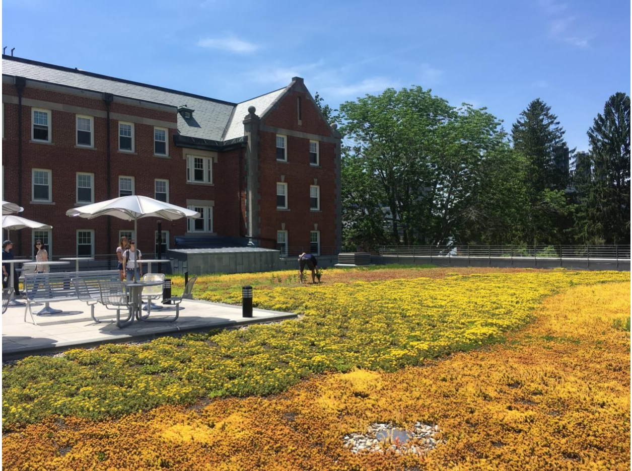
5 (green roof on Storrs Hall at the University of Connecticut, taken by Chester Arnold)
