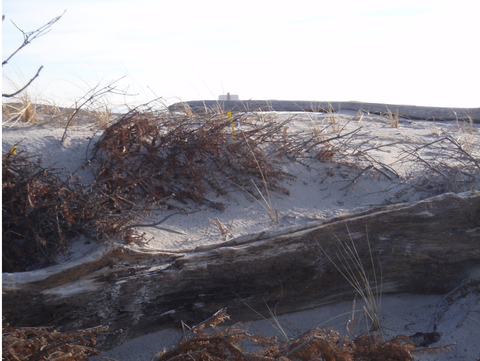
Figure 13b: Christmas trees used to trap sand at Waterford Beach, CT, via Connecticut Beach Dune Guide
