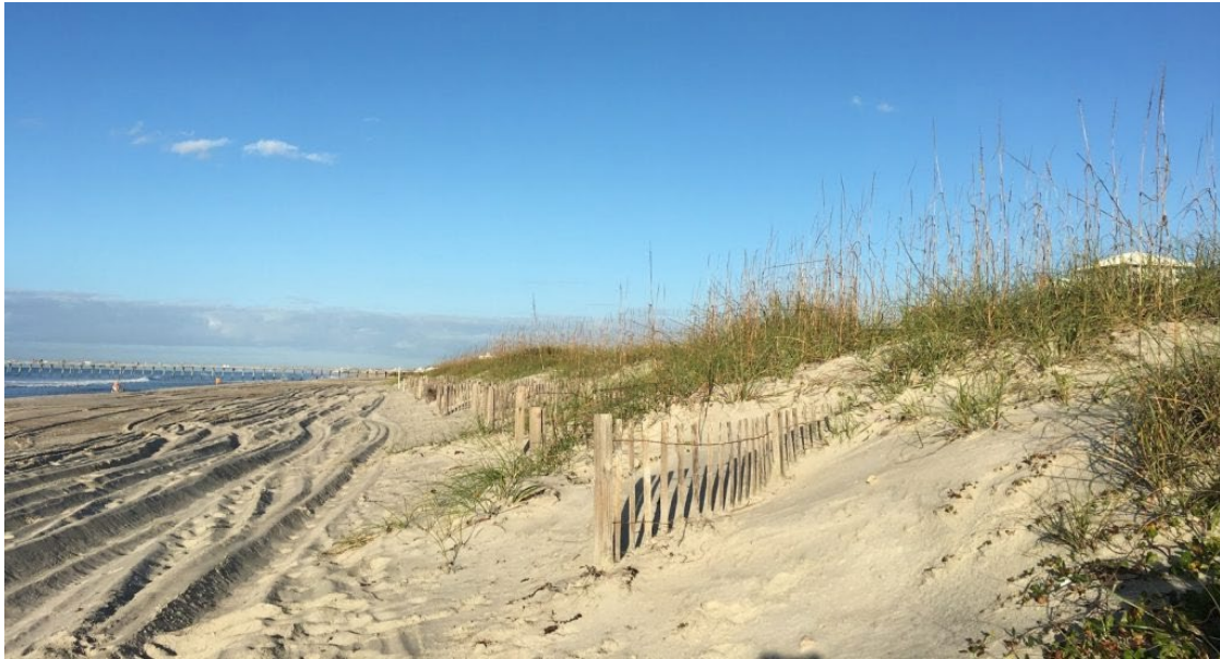
Figure 13a: Sand fencing along a dune in Bogue Banks, NC via NOAA
