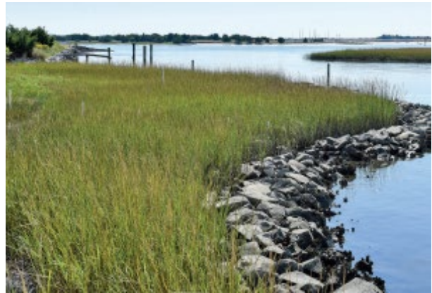
Figure 10a: Rock sill shoreline at NCCOS lab in North Carolina via NOAA
