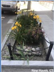
Bioswale captures and treats stormwater New Haven, CT
