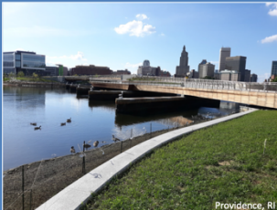
Bridge elevated to accommodate sea level rise Providence, RI
